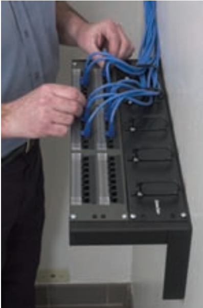
Wall-mounted Hub bracket with hub and cable manager installed
