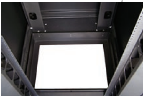
Sealed floor panel
